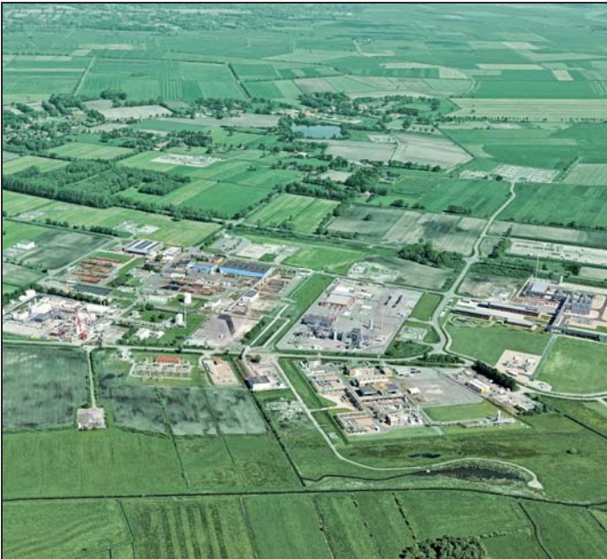
Kavernenanlage der STORAG ETZEL Cavern facility of STORAG ETZEL
