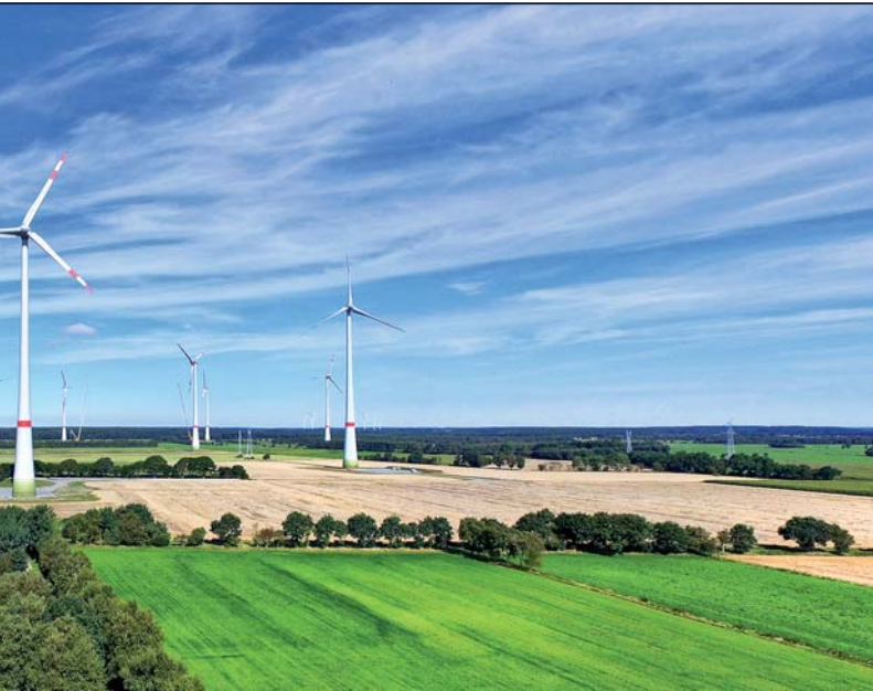
Whether offshore or on land: EWE is a pioneer in using wind energy.
